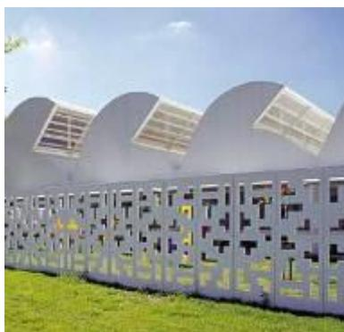
**Figura 03.b:** Hospital Sarah Rio – muro de painéis de argamassa armada. Fonte [www.skyscrapercity.com](http://www.skyscrapercity.com), foto my zoom.
