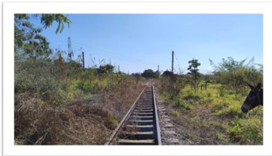
Figure 5 – Remnant of railway infrastructure
